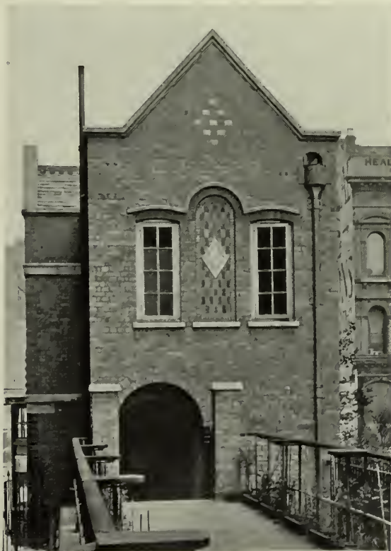
REAR VIEW, EXTENSION TO WHITEFIELD'S TABERNACLE, TOTTENHAM COURT ROAD, LONDON.
